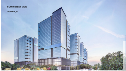
Southwest view of Tower_01, Phase_01, showcasing its 2.2 Million SFT space, standing tall at 159.5 meters with 7 basements.
